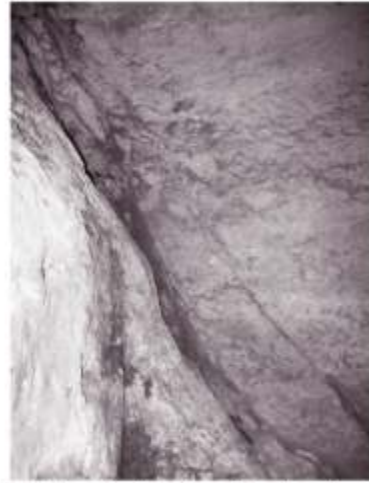
Fig.7a: Cave-V – Interior – Cracks in the Wall
