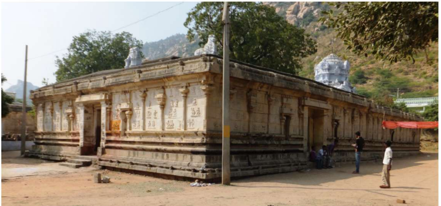
Fig.1 : Śiva temple at Penukonda, general view
